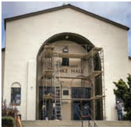
Grunke Hall exterior repair and painting
