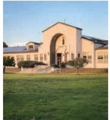
After new paint and solar panels—at no expense to MBA
